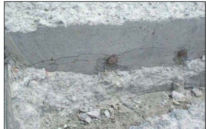
Cross-section of cracked pavement
