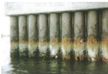
Photo-5.5.3 Corrosion conditions ①
