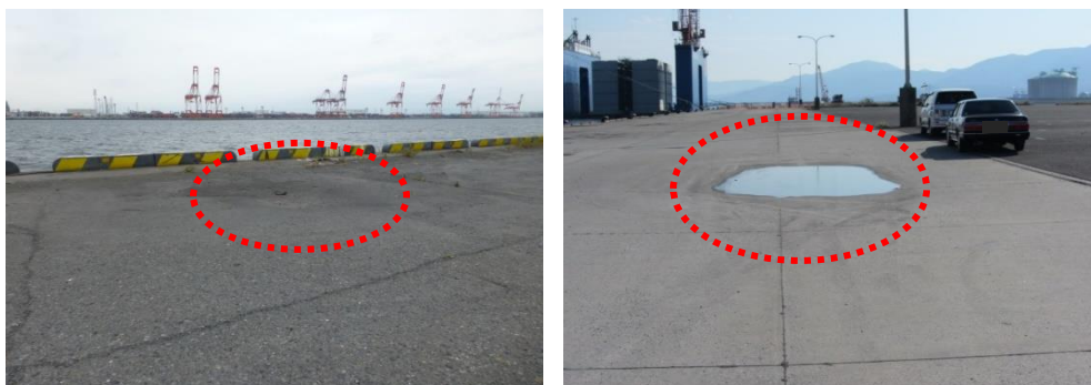
Photo-4.4.1 Example of a subsidence or collapse of the apron
