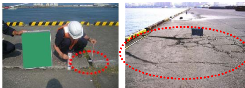
Photo-4.4.2 Examples of apron deformation
