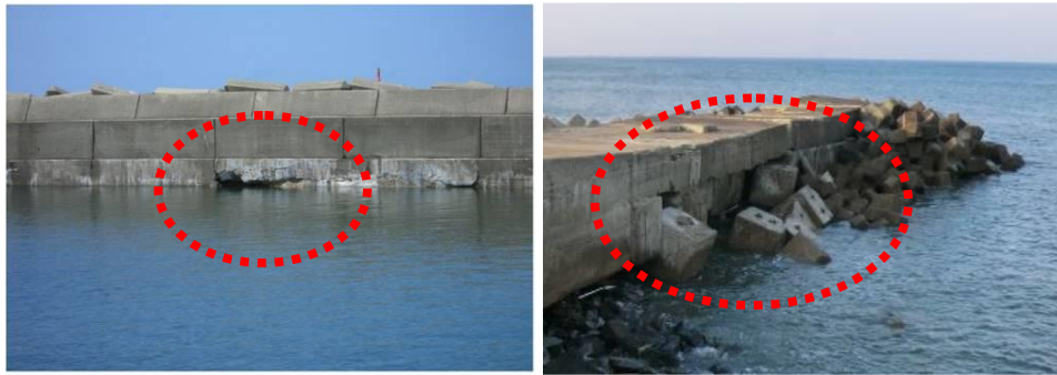
Photo-4.3.1 Deformations of concrete block-type breakwaters
