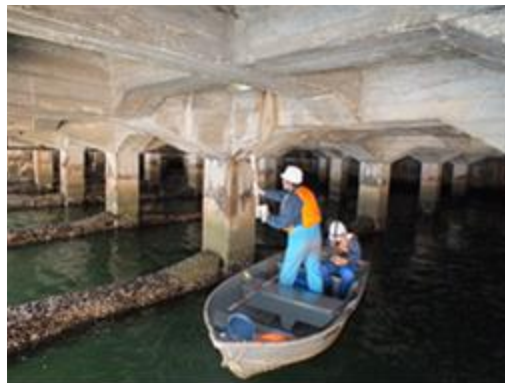
Photo-5.2.1 A visual inspection above sea level using a boat
