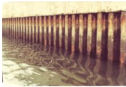
Photo-5.5.5 Corrosion conditions ②
