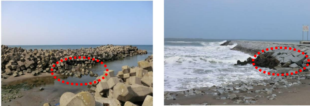
Photo-4.3.2 Deformations of rubble mound-type sloping breakwaters
