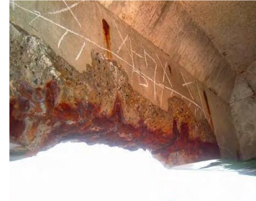
Photo-4.4.5 An example of deterioration on the bottom surface of a wharf superstructure
