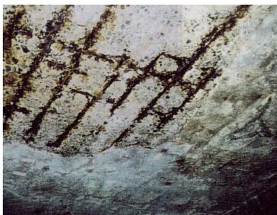
**Photo. 3.4.1.1 Corrosion of reinforcing bars in the superstructure (slab) of a pier
