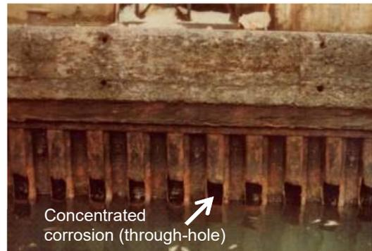
**Photo 3.4.1.2** Example of concentrated corrosion in steel sheet piles near the L.W.L.
