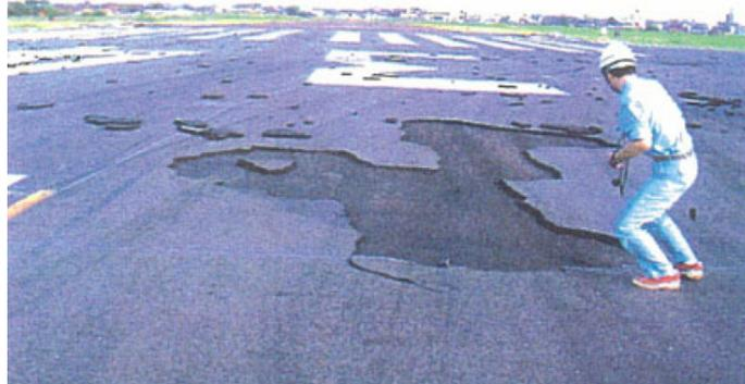
Figure 1 Slippage failure due to loss of bond at Nagoya Airport
