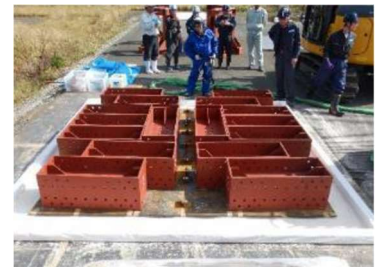
⑤ 鋼製山留設置
